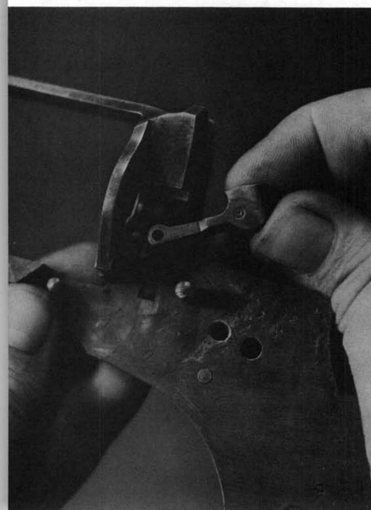
**16.** Tip the cartridge support block back until it clears the frame, then lift it off its post toward the left and remove it from the frame.
