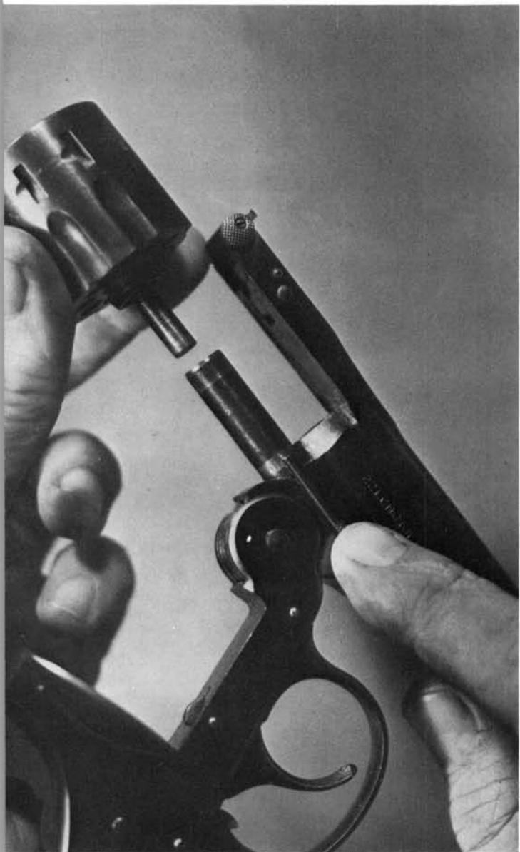
2. Grip the ejector post with smooth-jawed pliers and unscrew it counterclockwise (front view).
