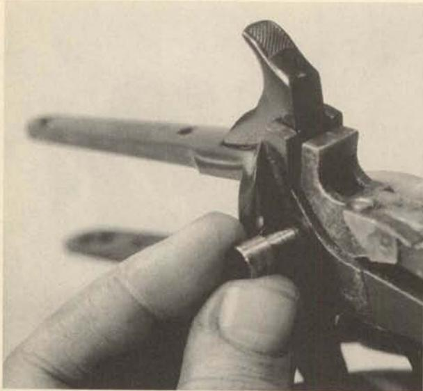
7. With a large diameter non-marring drift punch, push out the hollow hammer/cARRIER pivot toward the right.
