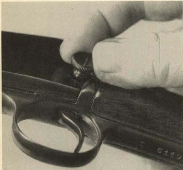
**2.** Set the hammer on the safety step, and move the rear portion of the gun off toward the rear.
