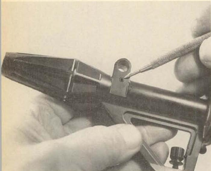
**21.** The twin magazine catches and their coil springs are pivoted and retained by vertical roll pins.
