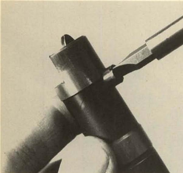
**5.** Release the firing pin and remove it toward the rear. The firing pin return spring may stay in its tunnel, and can be shaken out or extracted with a bent paper clip.
